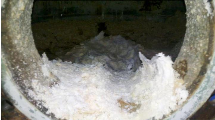
**Without HydroFLOW:** Limescale covers the bottom of the cylinder, and is very solid and compact (200kg total)
