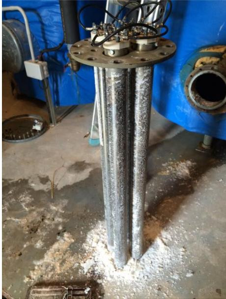
**With HydroFLOW:** Limescale was reduced by 95% It is light, delicate and turns into powder at a touch. The heater is operational.
