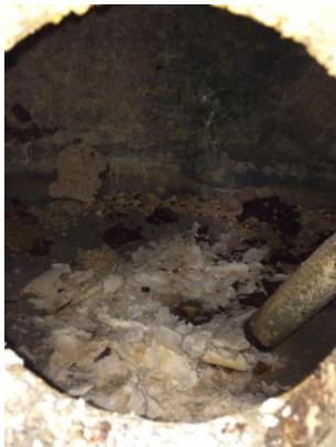
**With HydroFLOW:** Limescale was reduced (<10kg). It is light, fragile and transforms to powder when touched.
