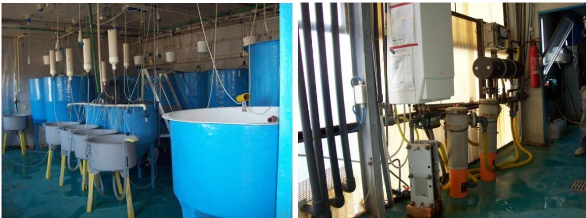
Figure 5: In these tanks (Right), new-born fish are placed to begin their growth. The Agriflow unit (right) protects the fish against bacteria, and also protects the heat exchanger against limescale.
