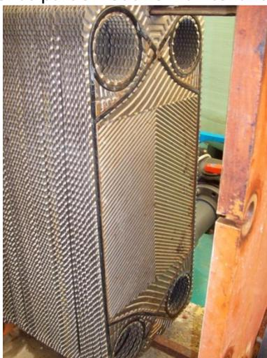
Figure 7: A heat exchanger protected against limescale by Agriflow. Instead of twice-yearly acid washes, the exchanger is hosed down once a year as part of routine maintenance.
