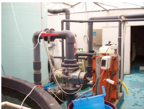
Figure 3: An Agriflow A100 unit installed before the water is transferred to the main fish tanks.
