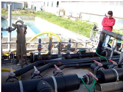
Figure 2: An Agriflow unit installed on the incoming water to the whole plant.
