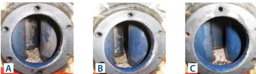
At a six month inspection, the hot water tank flues (A) were scale free but covered by light talc (an expected result of breakdown of existing limescale). The talc easily wiped off with a cloth (B and C).
