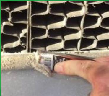
90 days into the demonstration, deposits inside the tubes and on the fill media did not increase after chemicals were reduced and the water concentration cycles were increased. Hard scale deposits began to soften and could be removed easily.
