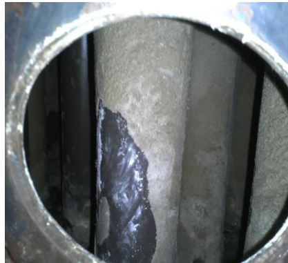
After 4 weeks - Limescale became softer and was easily flaked off
