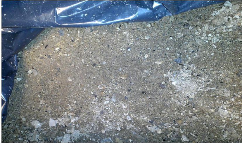
Scale that came off the heater tubes
