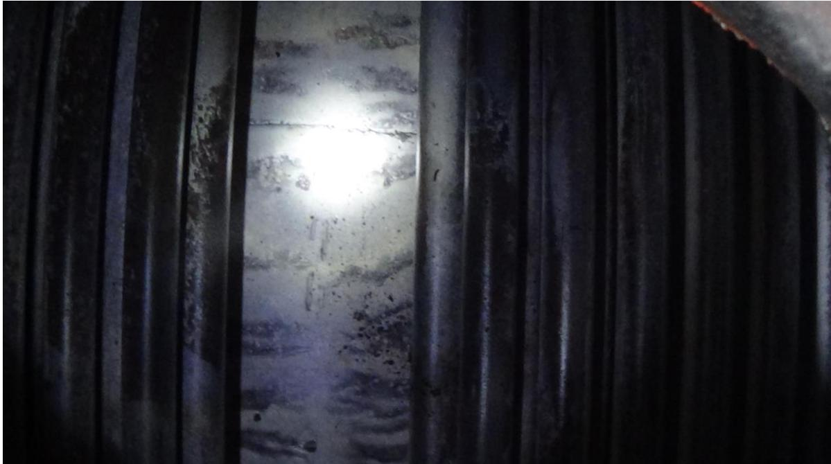
The boiler tubes were found to be completely clear of scale – cleaner than they had been immediately after cleaning, indicating that the unit had removed existing scale. The surfaces of the boiler shell were also clear of hard scale, with just a fine powdery deposit remaining. There was no need for the difficult descaling that previously took 3 days.
